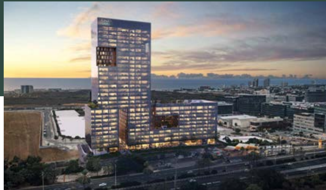
South Gate, Herzliya Pituah Status: Under Construction
